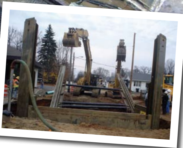
Left: The excavation is in a very tight spot in the right-of-way of Twyckenham Drive in a residential area of South Bend Indiana, eliminating the possibility of trench shields or sloping. Instead, Woodruff & Sons, Inc. Contractors installs a Slide Rail System from Efficiency Production, just a few feet from existing structures.
