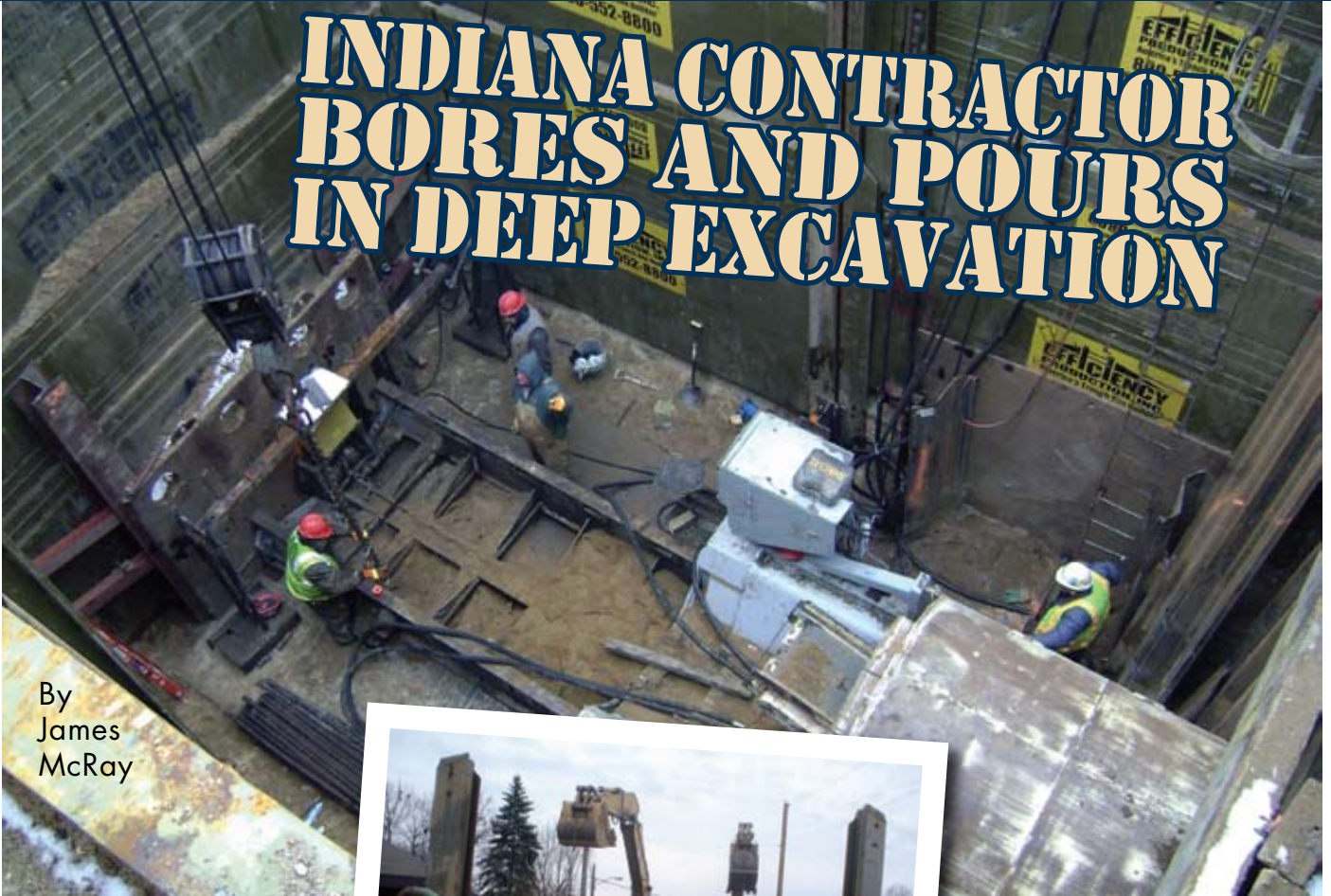
Above: The sheeting was perfect for boring the 72-inch-diameter pipe, which was handled by boring specialists L.J. Keefe, out of Mt. Prospect, Illinois.
